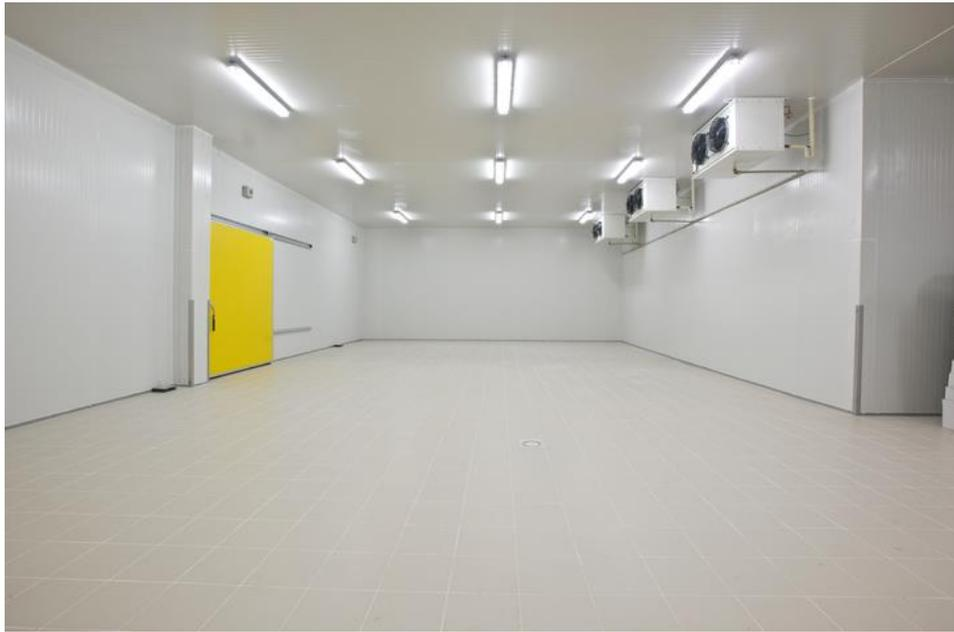
**Figure 1: New walk in coolroom with three evaporators.**
